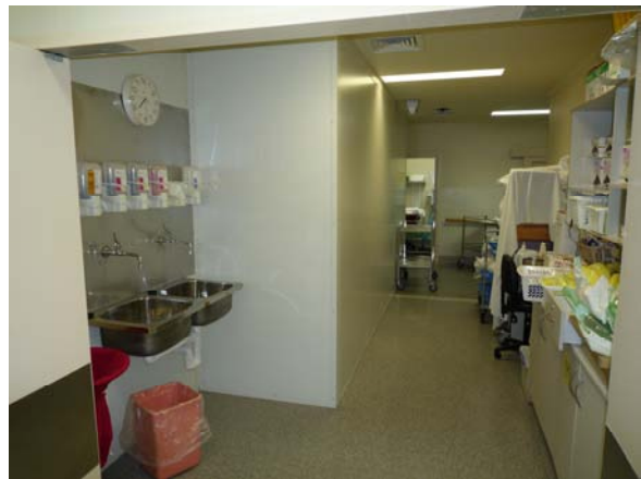
The new temporary wall and scrub troughs seen from OR 5
